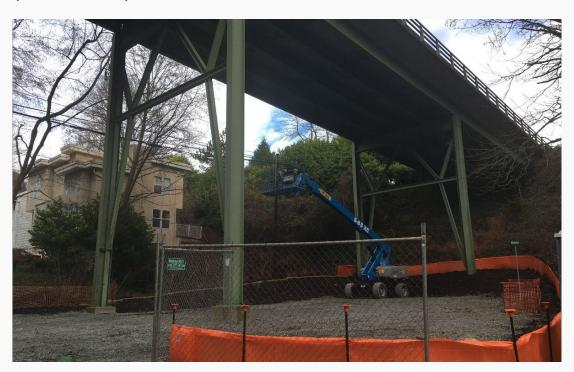
Currently construction on the W Howe St Bridge is suspended while we wait on the fabrication of the plates. Work is anticipated to resume as soon as early March. Access to the bridge will remain open throughout the suspension. We will be in touch with the nearby community to share details before work resumes.
